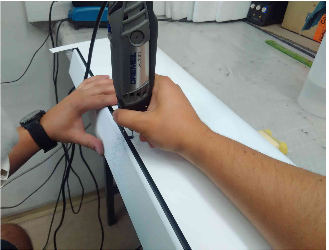
Cutting the pieces
