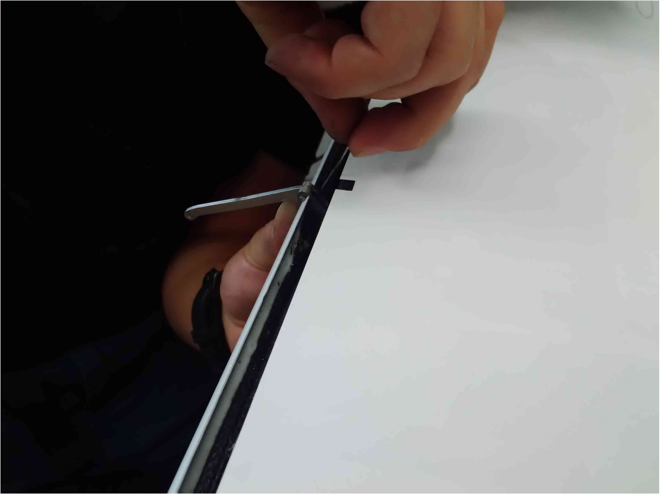
introducing the glue with a tool
